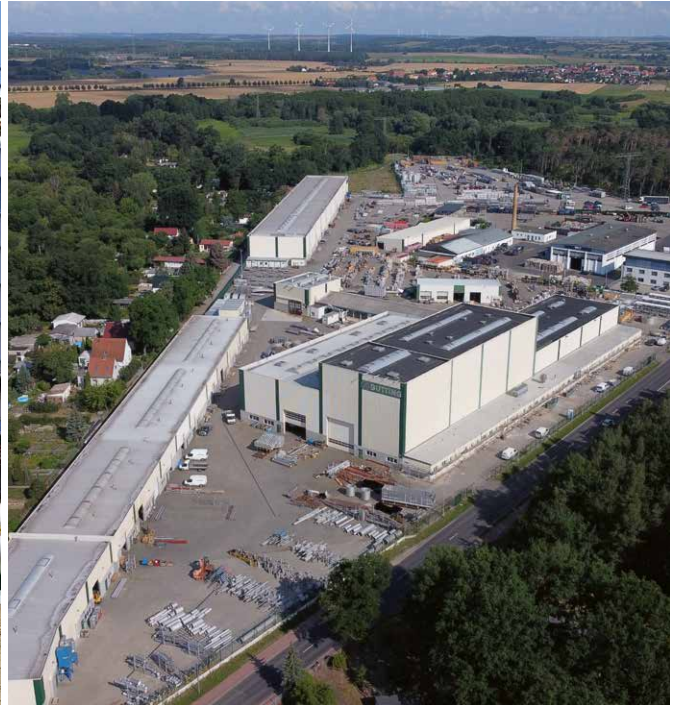
BUTTING in Schwedt, Germany
