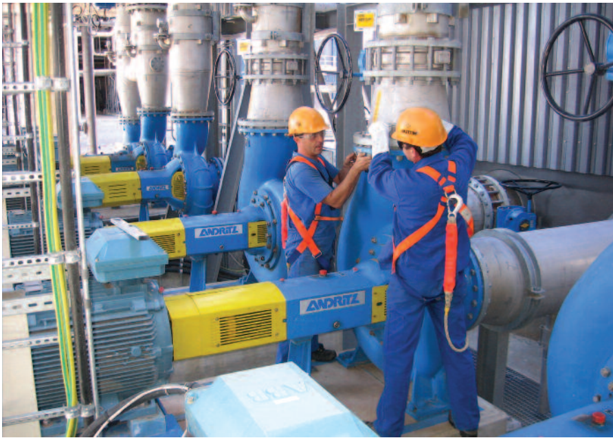
Worldwide installation of pipelines and vessels for selected industries including the paper and pulp industry and bio-energy technology.
