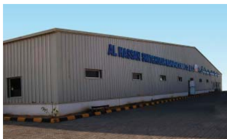
New Switchgear Manufacturing Facility - Buraimi
