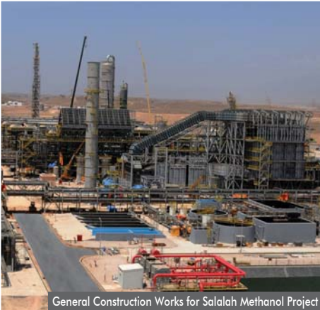
General Construction Works for Salah Methanol Project
