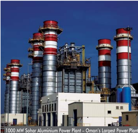
1000 MW Sohar Aluminium Power Plant - Oman's Largest Power Plant
