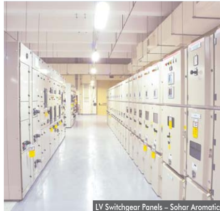
LV Switchgear Panels - Sohar Aromatics
